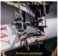
At this point, the area will likely become crammed with supports and clamps, so compact finger clamps are best, such as the small steel ones shown in the photo below.
