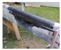
plastic kitchen wrap around the whole mast section to bed this new material firmly to the initially flexible nose, which will become stiffer and stiffer with each layer, until the final layer is flush with the original mast .... checked with a long metal straight edge.
