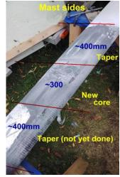
To be level, the surface should be lightly sanded and then faired using lightweight microballoons.
