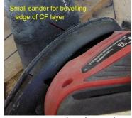
100 times the wall thickness, so if its 2.5 mm at the nose, that mean tapering it not less than 250mm. (On the sides, that distance will be more like 400mm so work with a straight edge in one hand to be sure the skin taper is gradual, straight and fair).
